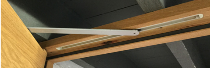
concealed overhead door closer (optional)
